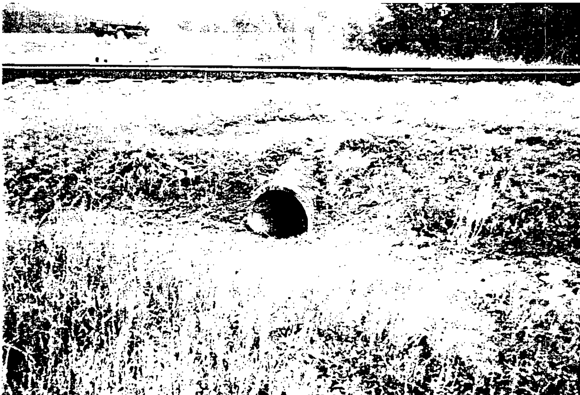
Figure 8. Photograph of the culvert connection to the drainage swale at the USAC railroad track (December, 1992).
