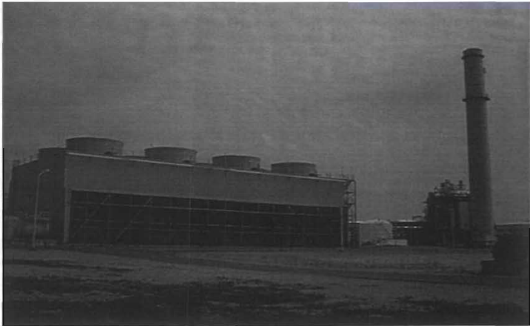
Photo 1. Distant View - Cooling Towers
