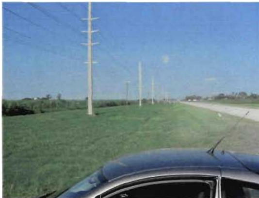
Figure 6 - View towards West
