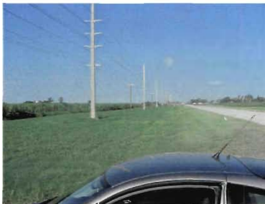
Figure 6 - View towards West
