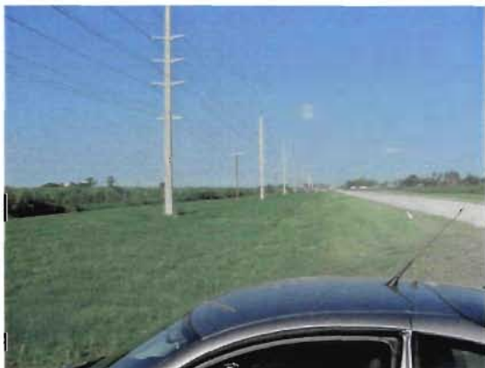
Figure 6 - View towards West
