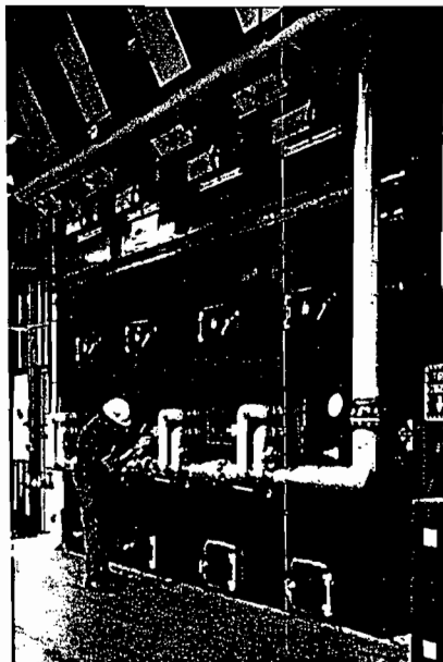
◀ Zurn stationary water-cooled-grate spreader stoker allows intermittent zoned cleaning of grates in a 120,000 lbs/hr unit at a Georgia paper plant.
