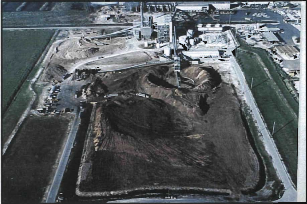
Figure 3.2-3a. NHPP Wood and Bagasse storage and handling.
