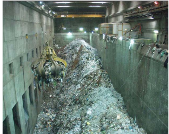
Figure 10 - Refuse pit at Brescia facility, Italy
