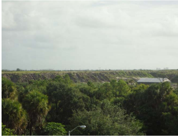
Figure 3 – Existing SWA Landfill
