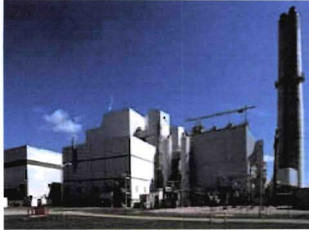
North County Resource Recovery Facility
