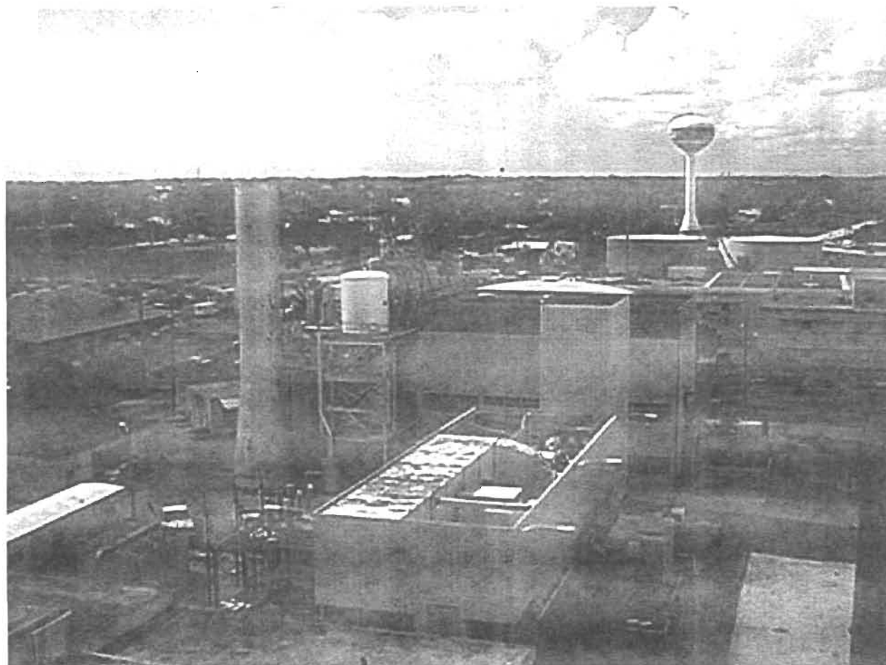
Photo 1. Aerial View - Stack and Building Location for Unit GT-I
