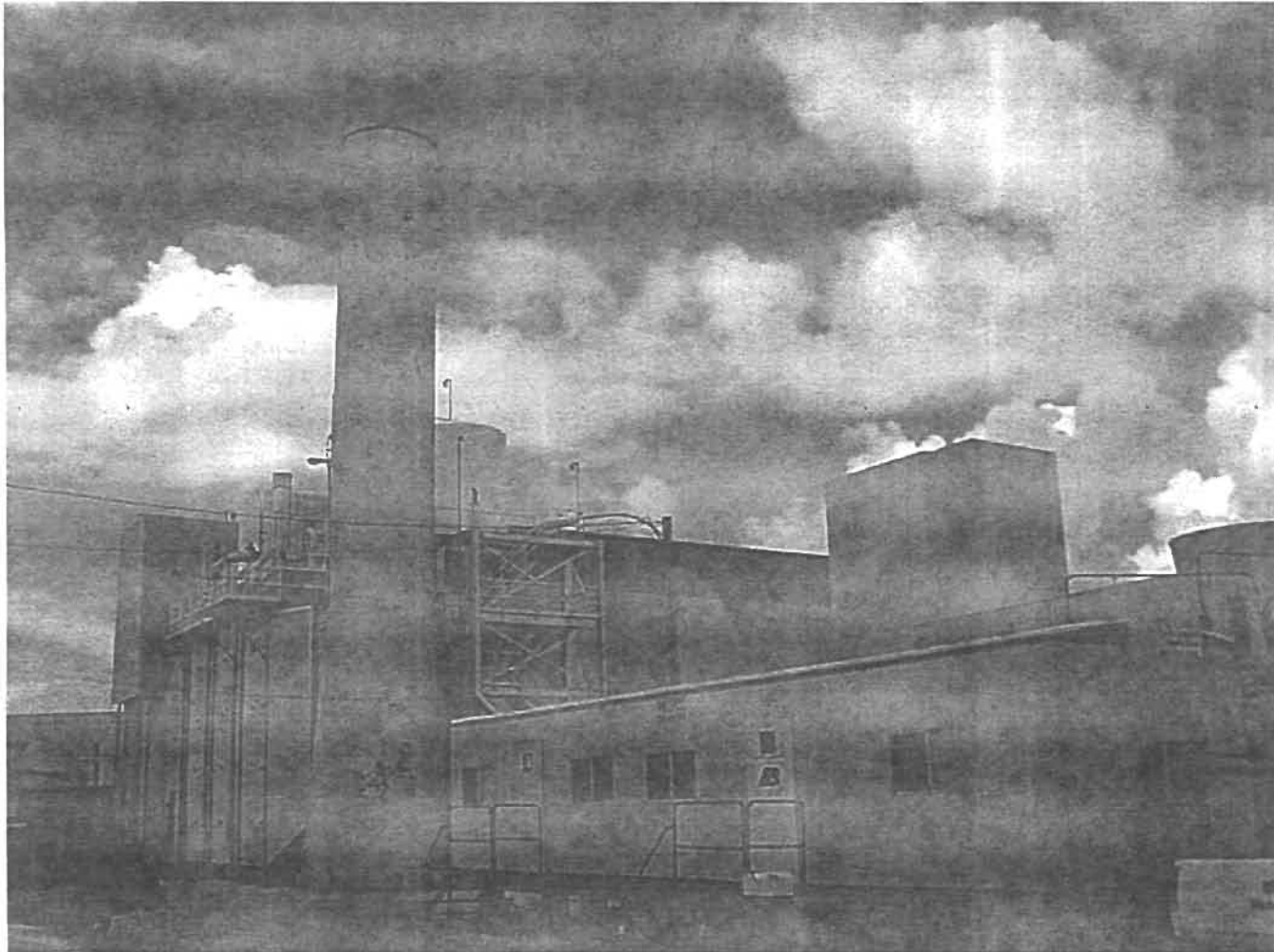
Photo 1. Outside View - Stack and Building Location for Unit GT-2/S-5
