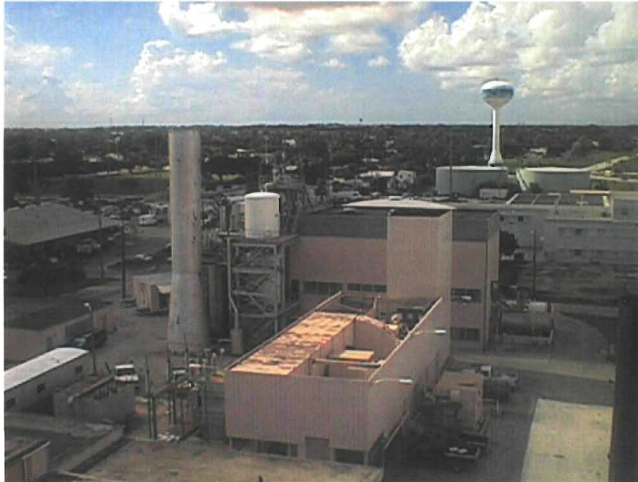
Photo 1. Aerial View - Stack and Building Location for Unit GT-1
