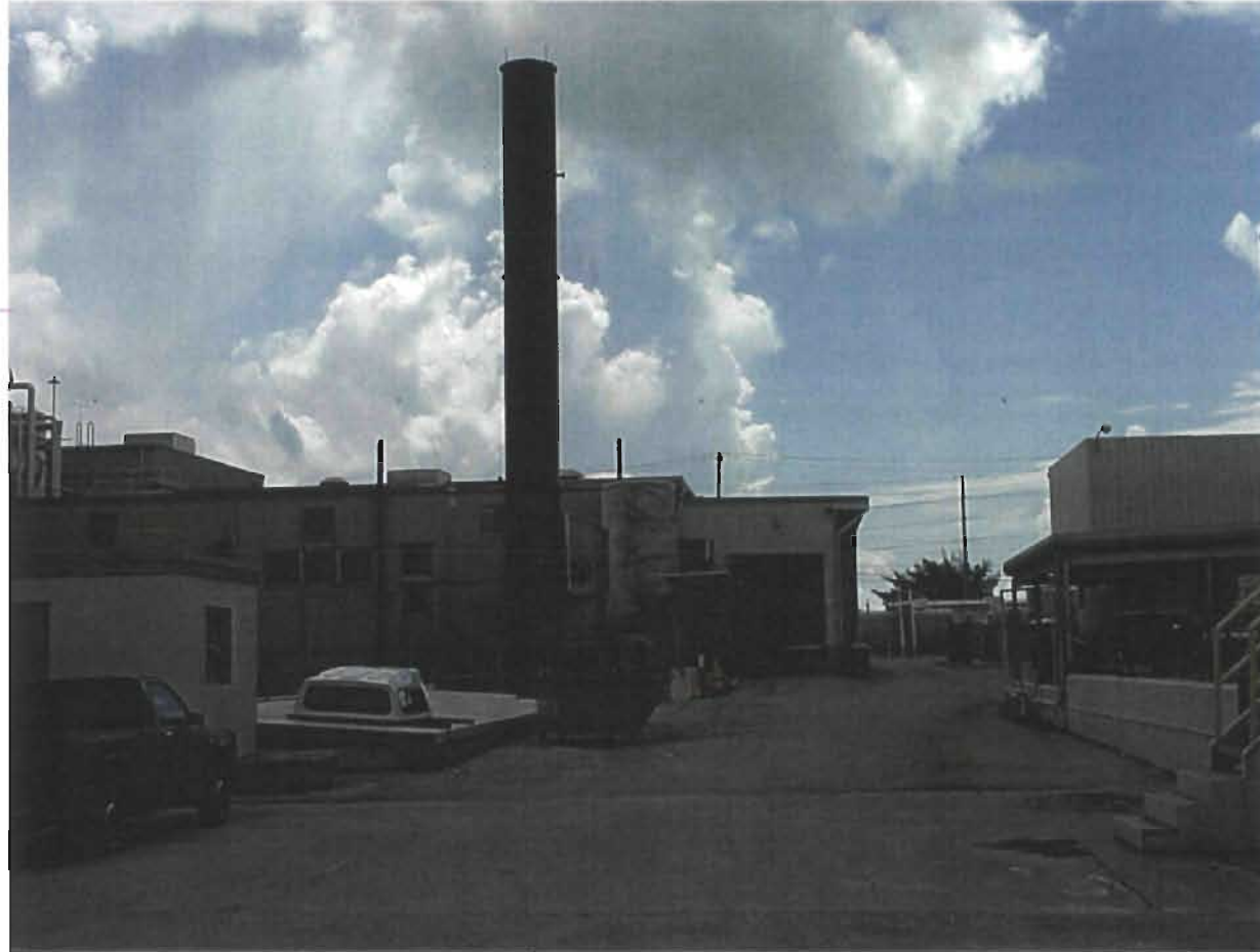
Photo 1. Outside View - Stack and Building Location for Unit S-1
