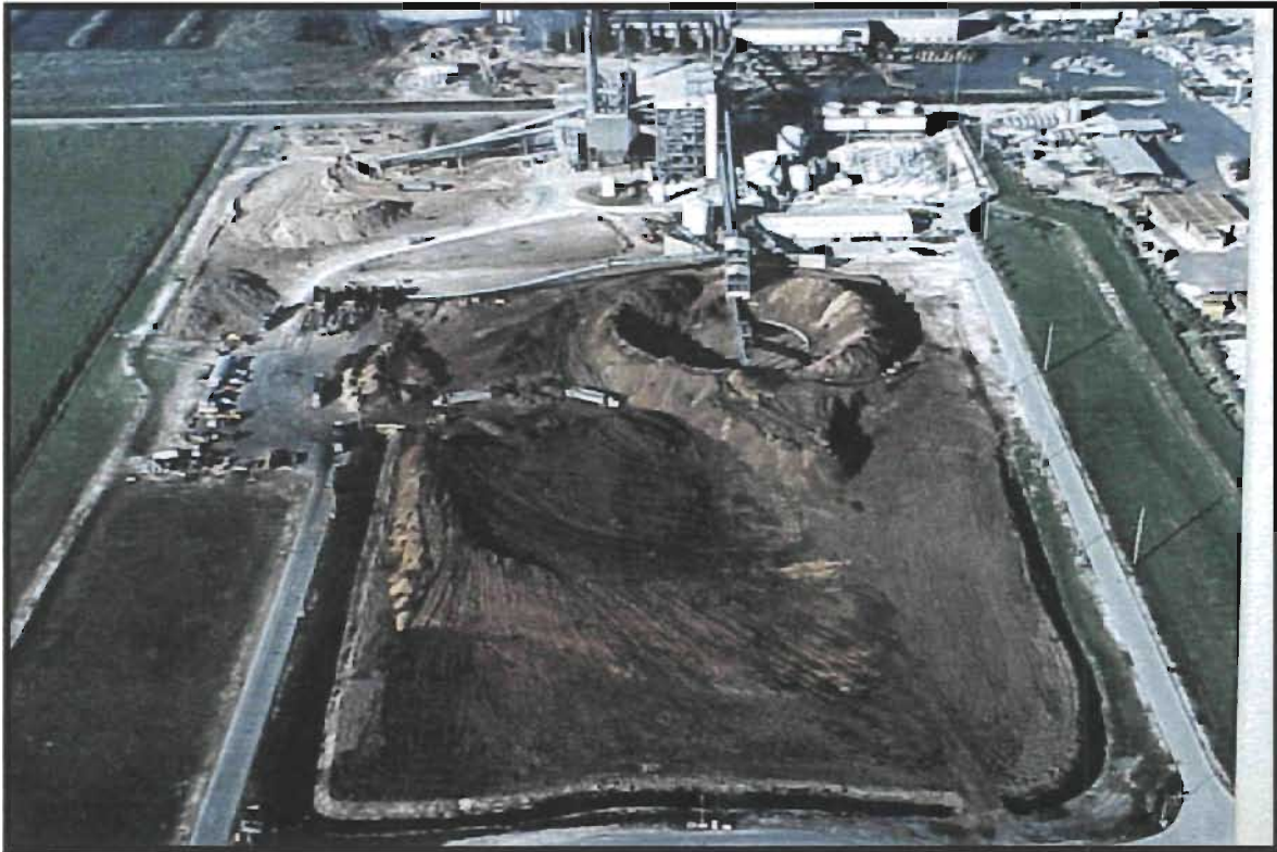
Figure 3.2-3a. NHPP Wood and Bagasse storage and handling.
