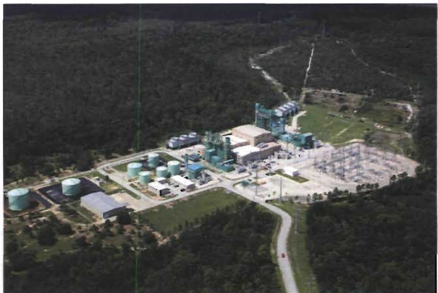
Figure 2. Aerial View of CIPP Units 1, 2 and 3 (left to right)
