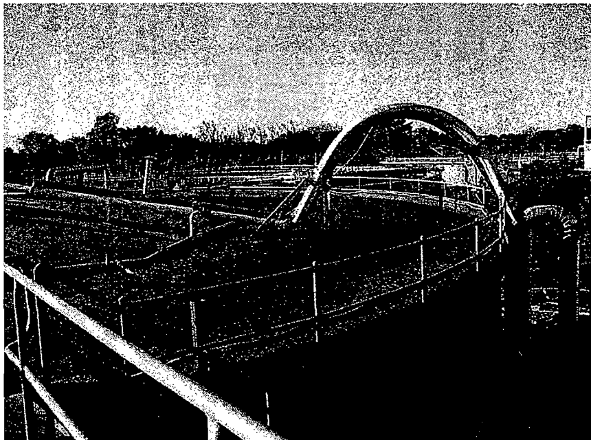
Photograph 1: Digester No. 6 Gas Collection Piping
