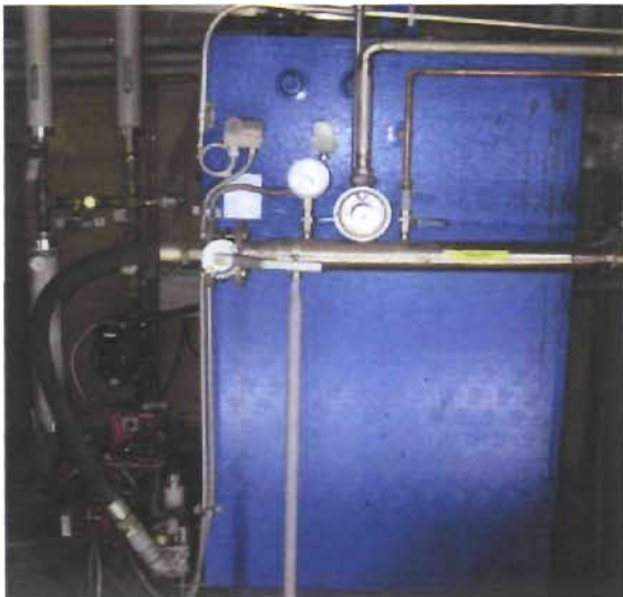
Figure 6: Oulu Municipal Solid Waste Management's Rusko landfill site 250kW central heating unit. In 2005, 874MWh of LFG was used for space heating at Rusko landfill site.
