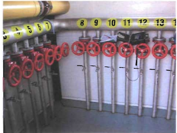
Figure 4: Gas Measurement Lines (20 lines). CH 4 , CO 2 , and O 2 flow and composition measurements are taken from each line once or twice a month.
