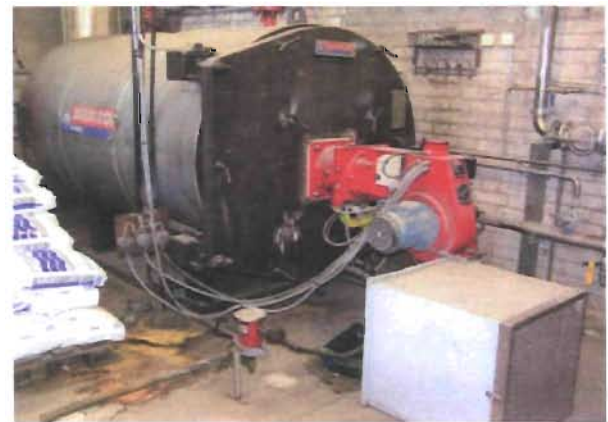
Figure 7: Paroc Ltd. Space Heating Unit. Paroc stone-wool factory, an intensive energy user, utilizes LFG as the main fuel in its operation - stone is smelted in manufacturing insulation used for construction purposes.
