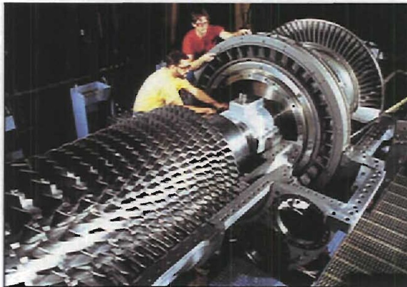
Figure 4 – Internal View of GE 7FA. (GE Website)
