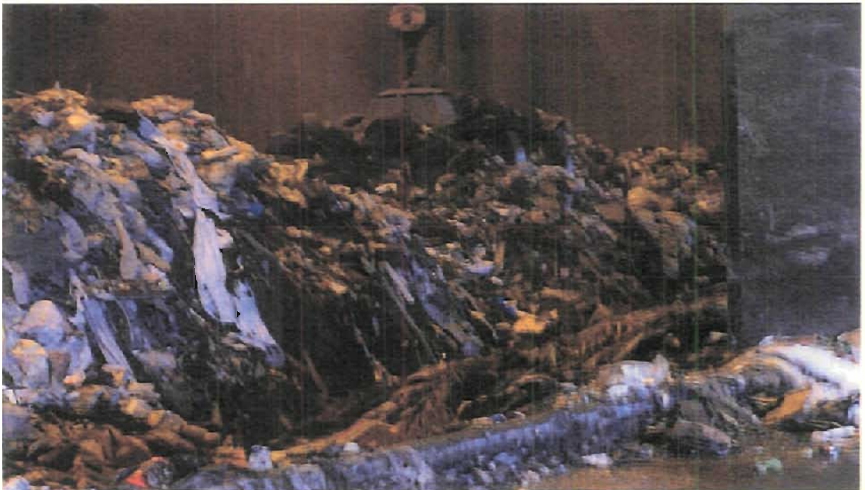
Waste Storage Bunker and Crane Grapple
