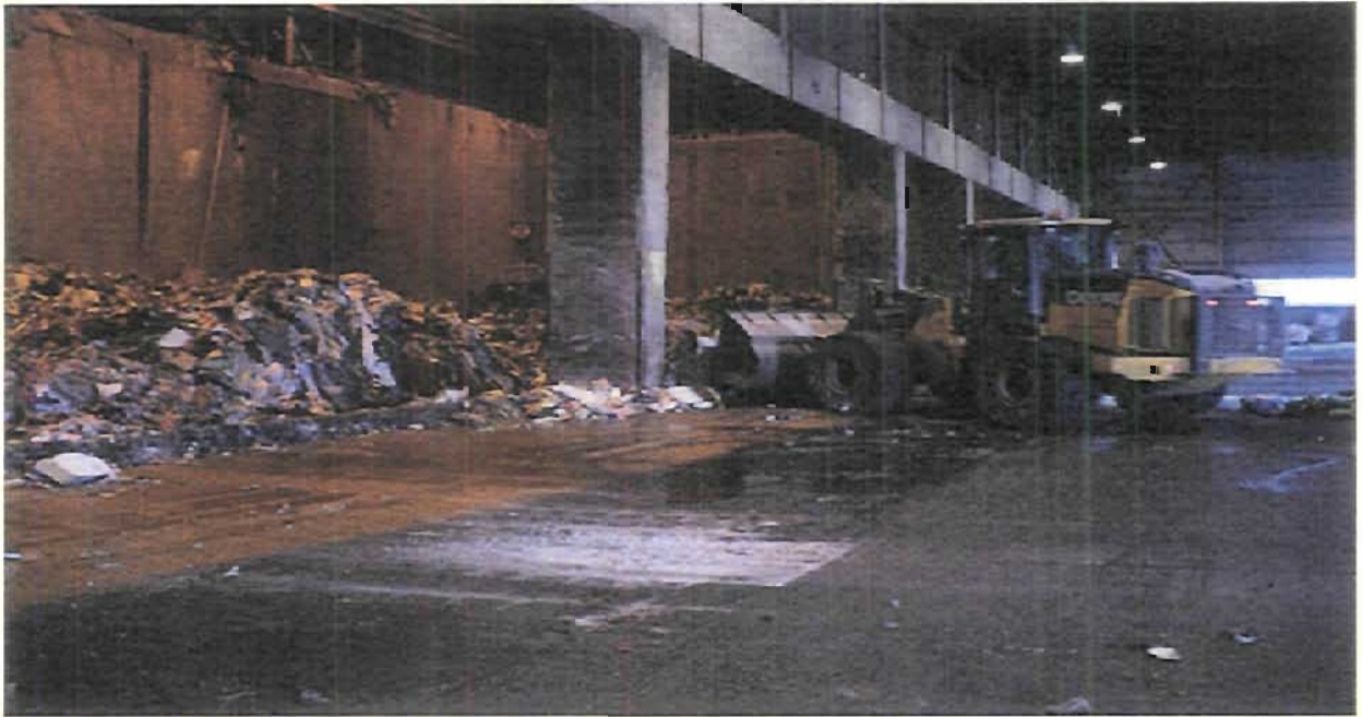
Tipping Floor and Waste Storage Bunker
