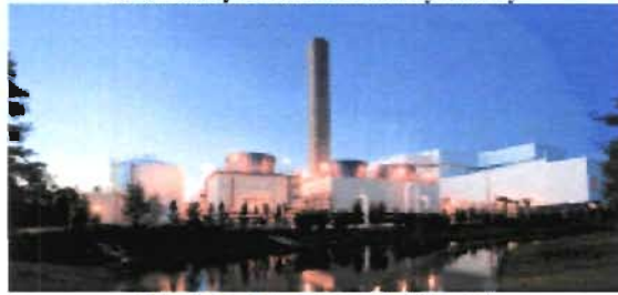
Lee County Resource Recovery Facility
