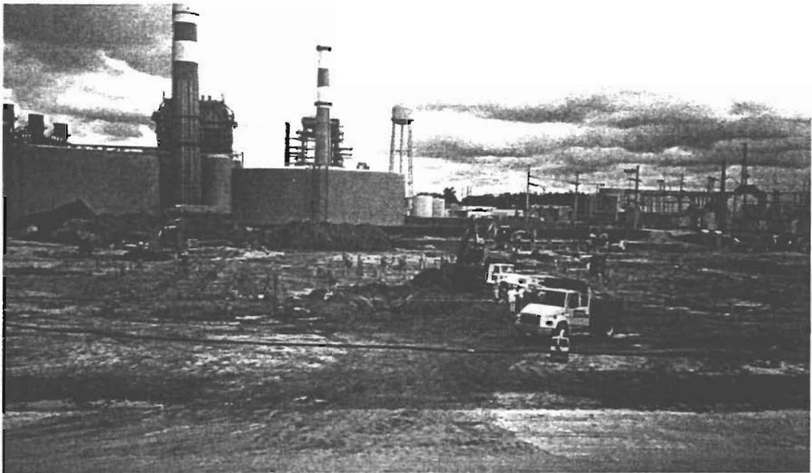
Fort Myers Plant - Simple Cycle Peaker Project - June 24, 2002
