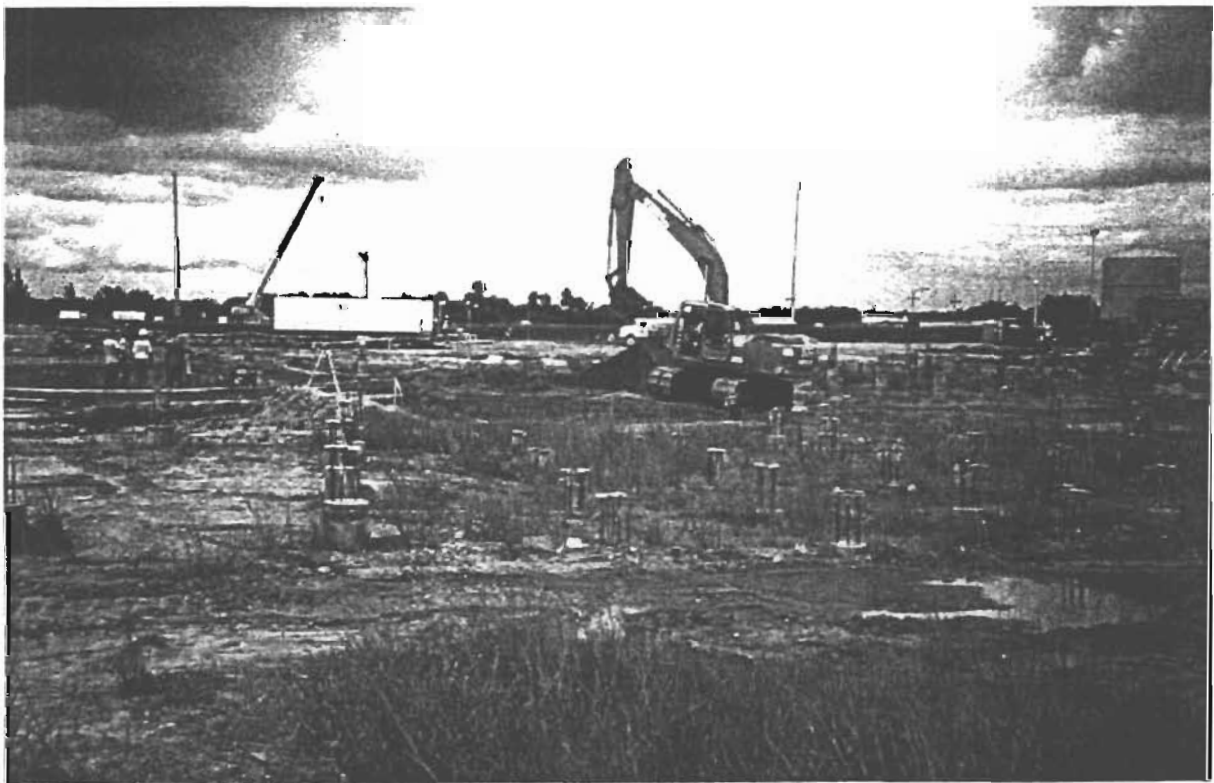
Fort Myers Plant - Simple Cycle Peaker Project - June 24, 2002
