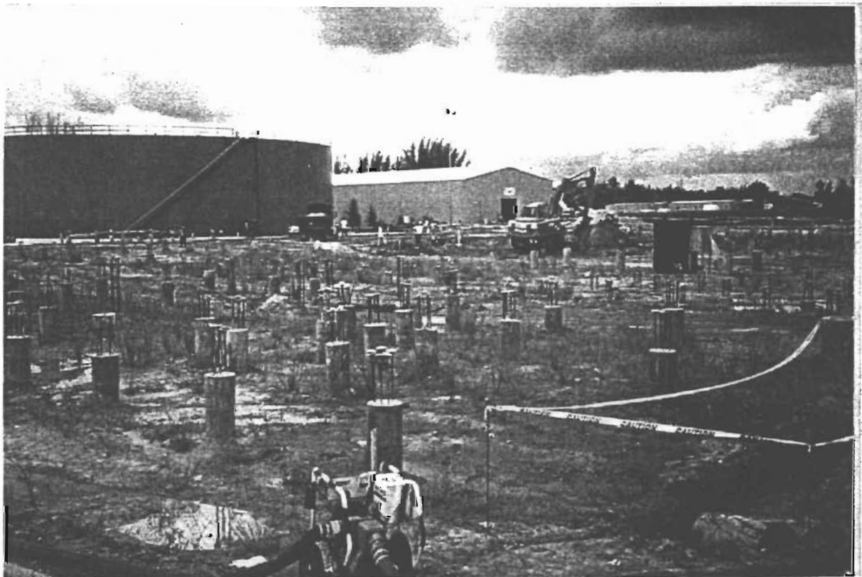
Fort Myers Plant - Simple Cycle Peaker Project - June 24, 2002
