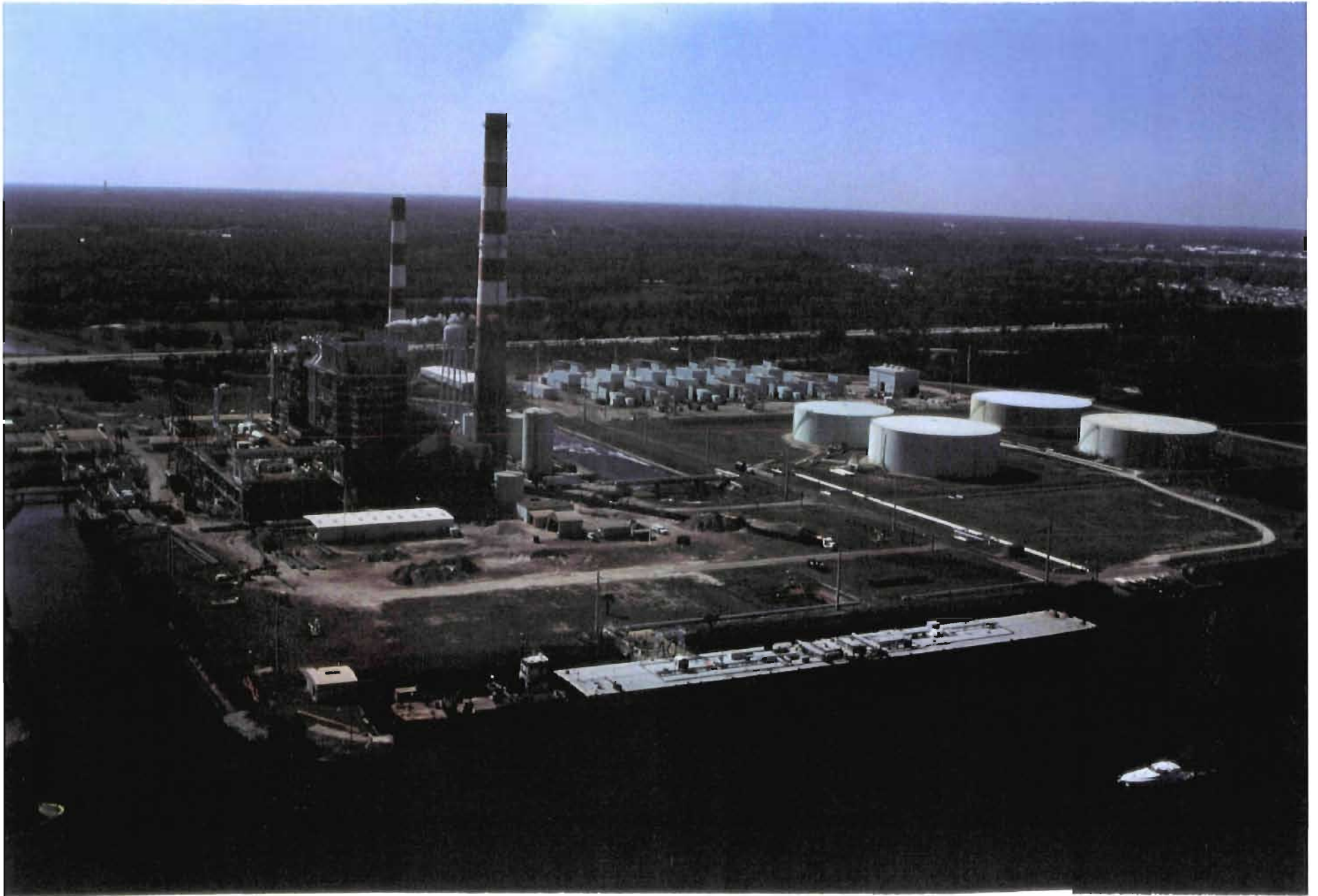
FORT MYERS PLANT VIEW FROM CALOOSAHAATCHEE RIVER
