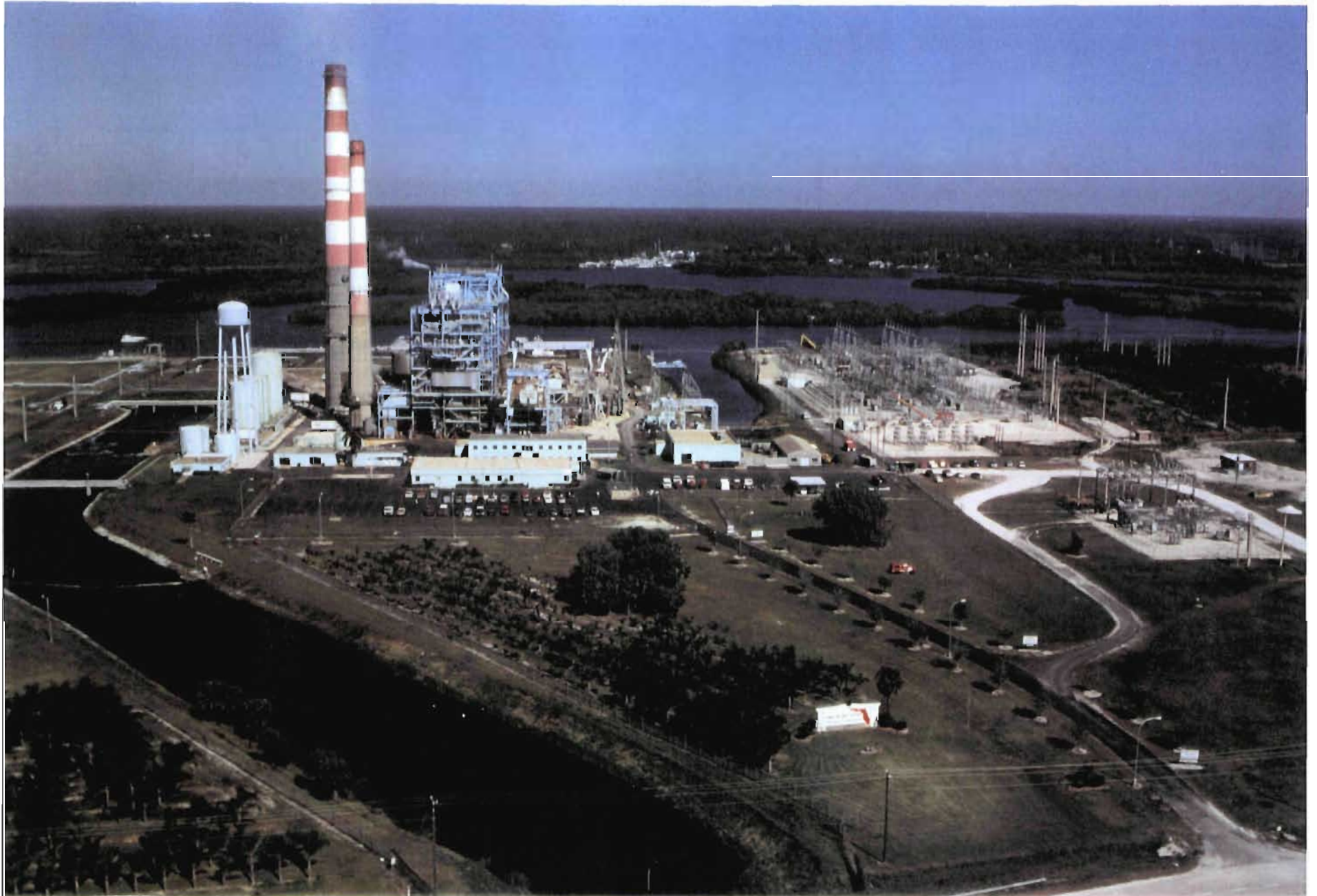
FORT MYERS PLANT VIEW FROM STATE ROAD 80
