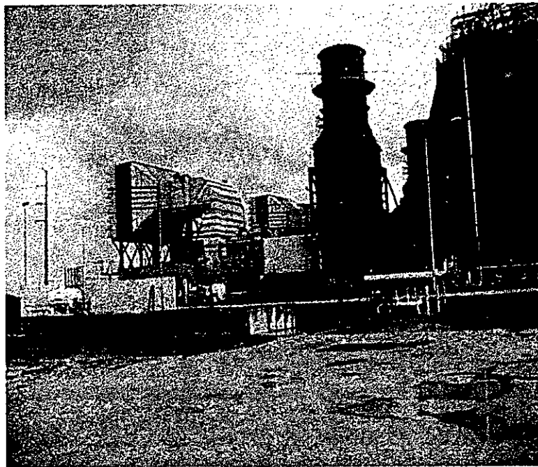
Figure 3 – View of the Combined Cycle Combustion Gas Turbines
