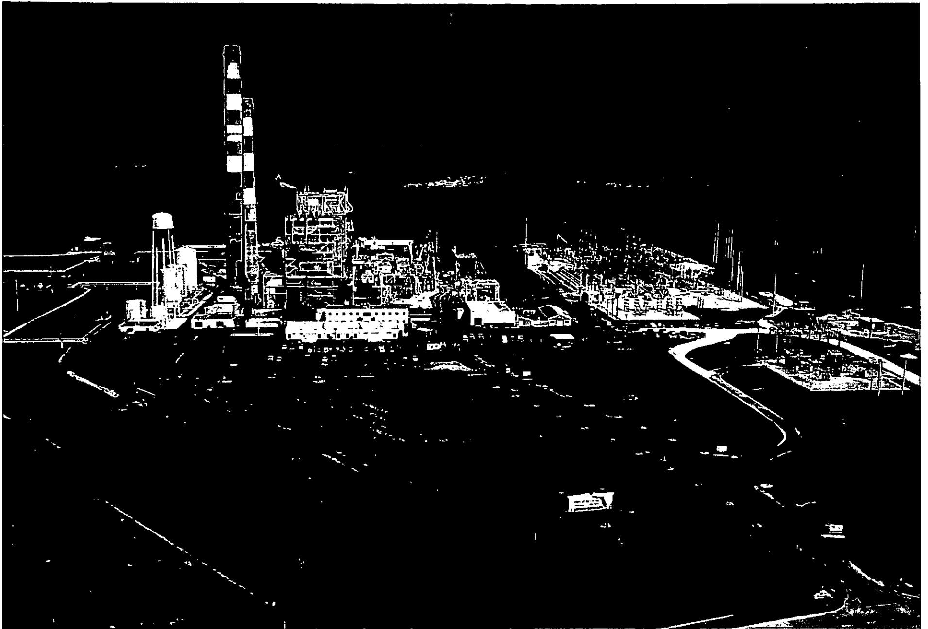
FORT MYERS PLANT VIEW FROM STATE ROAD 80
