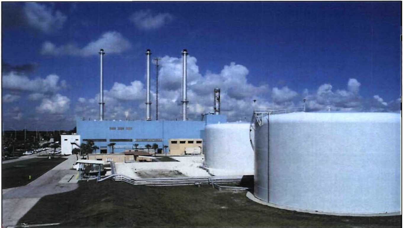
Photo 2. Profile View of Vero Beach Municipal Utilities
