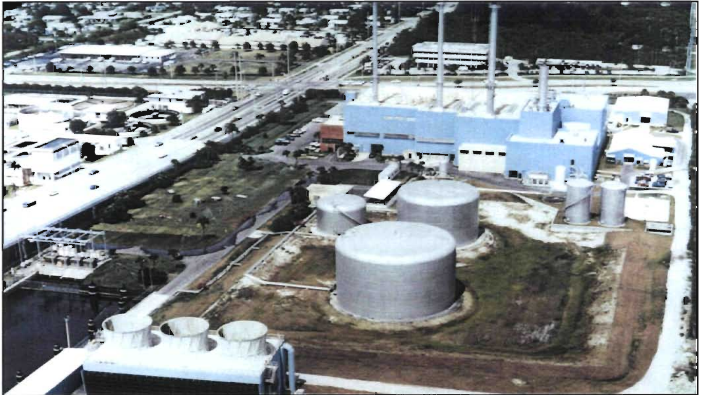
Photo 1. Aerial View of Vero Beach Municipal Utilities
