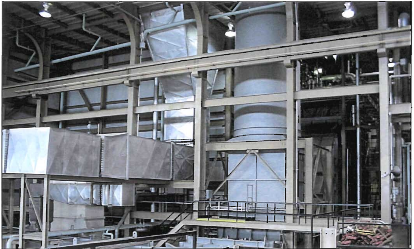
Photo 5. Internal View of Unit 5
