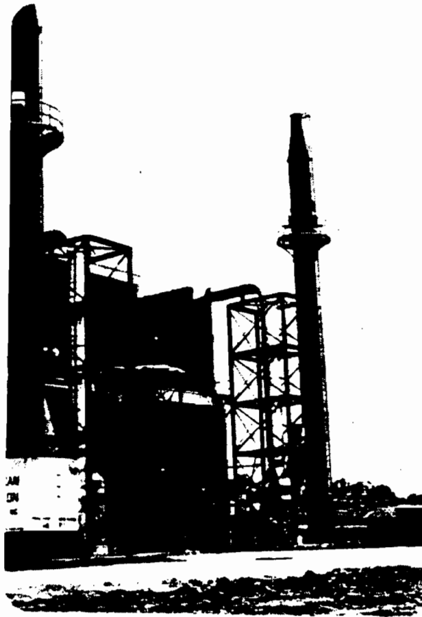
Photograph of Sampling Point 1, Stack
