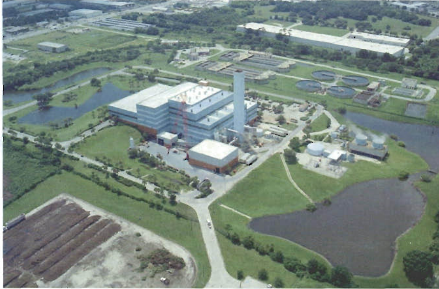
Hillsborough County Resource Recovery Facility
