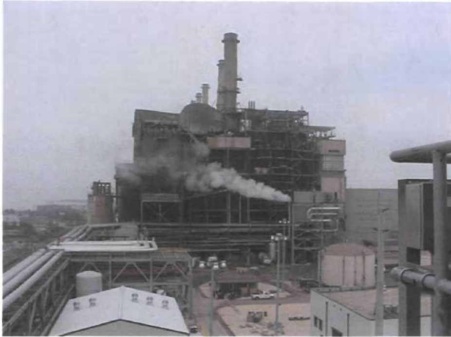
Picture #1. TECO-Gannon Plant looking west {the old plant}
