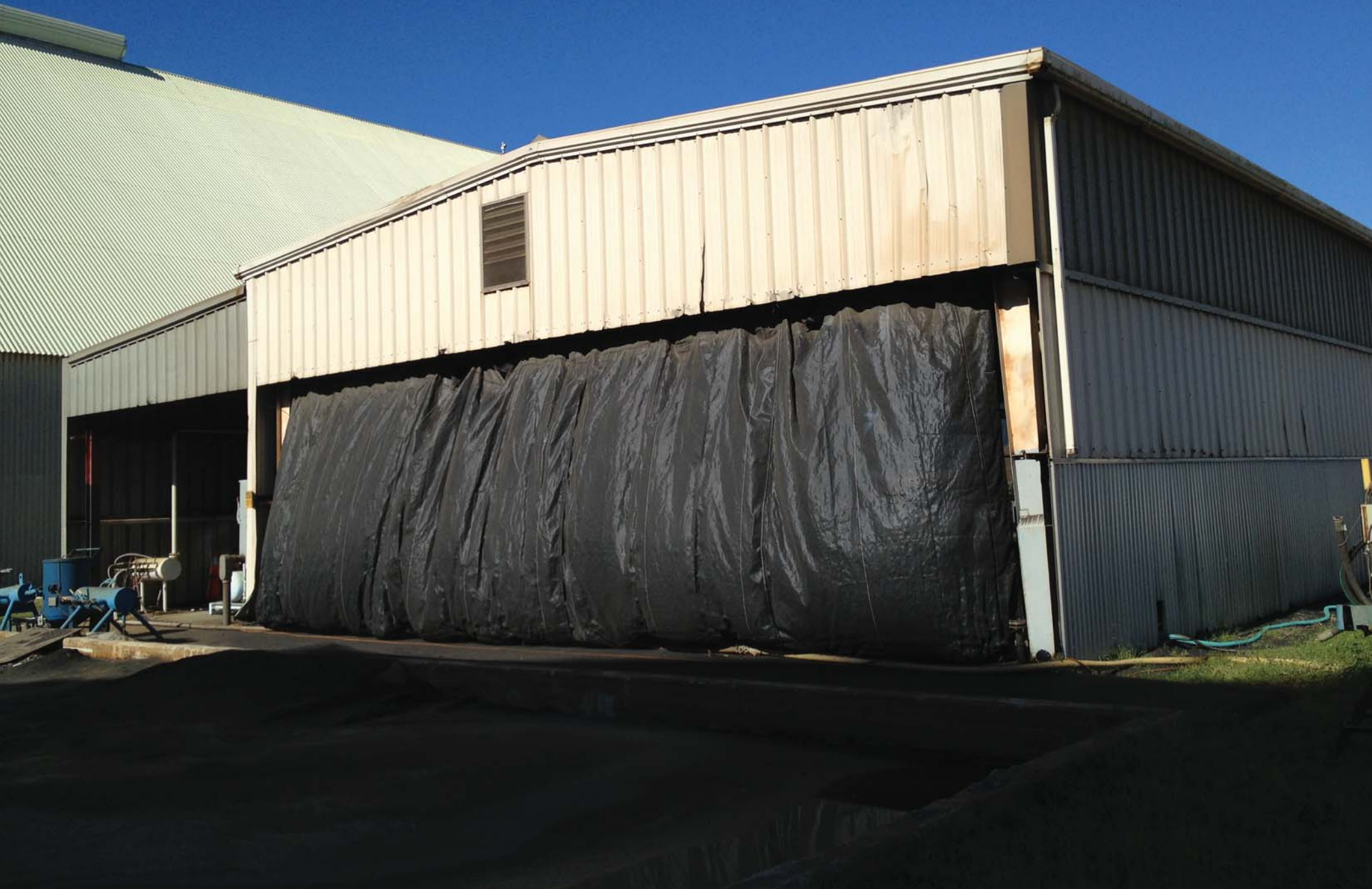
Response 4 - Existing Abrasive Blasting Building
