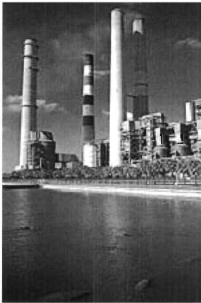
TAMPA ELECTRIC COMPANY BIG BEND STATION
