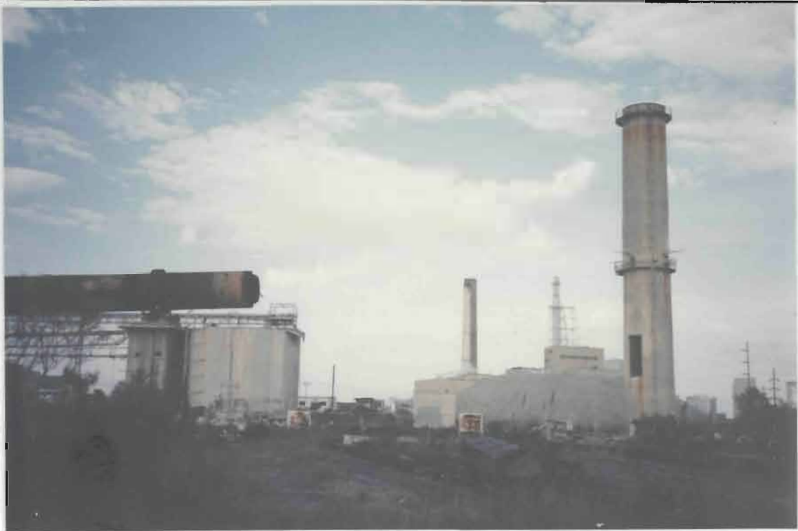
I. Side view of kiln showing space between stack and feed end of kiln where ESP was before removal. Note seal extension (smaller diameter) on kiln demonstrating that kiln remains at full length.
