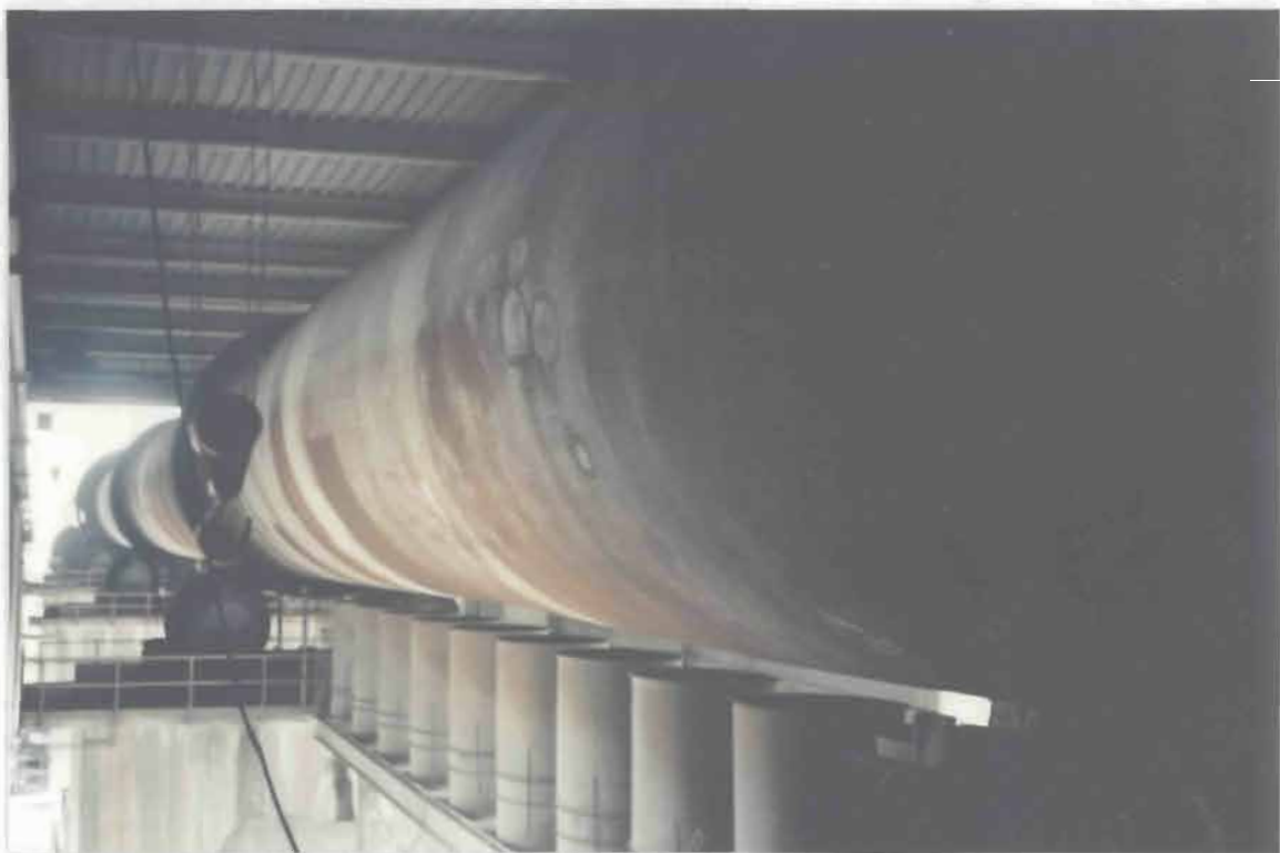
II. Axial view of kiln taken from burner floor looking uphill.
