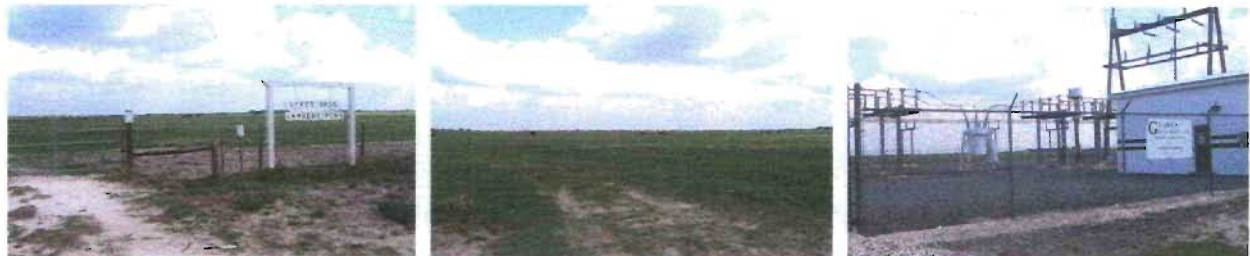
Figure 2 - Entrance to Proposed HEF Site, View of the Proposed Site, Adjacent Electric Substation.
