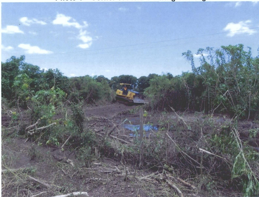
Photo 1 – Corner of Field 1 during clearing
