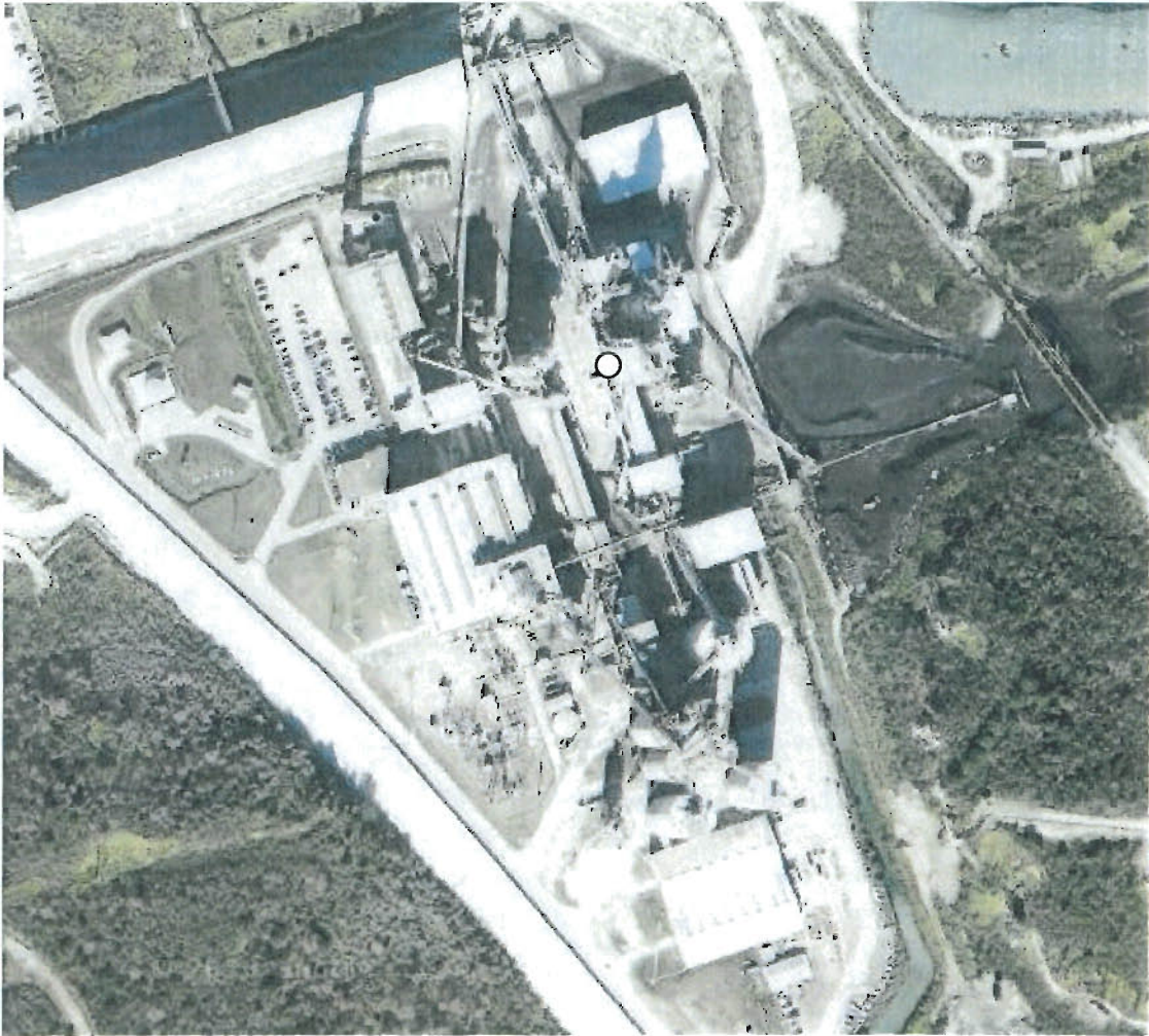
FIGURE 9. LOCATION OF THE PROCESSING AREA NEXT TO THE KILN 2 PRECALCINER.
