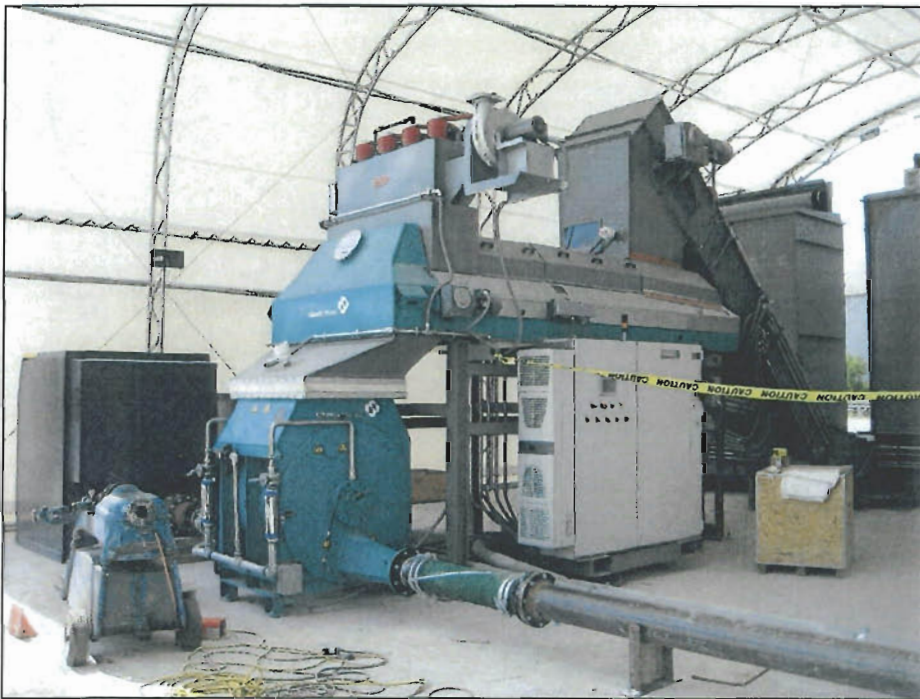
FIGURE 7. PNEUMATIC BLOWER FROM METERING SYSTEM TO INJECTION PORTHOLE.
