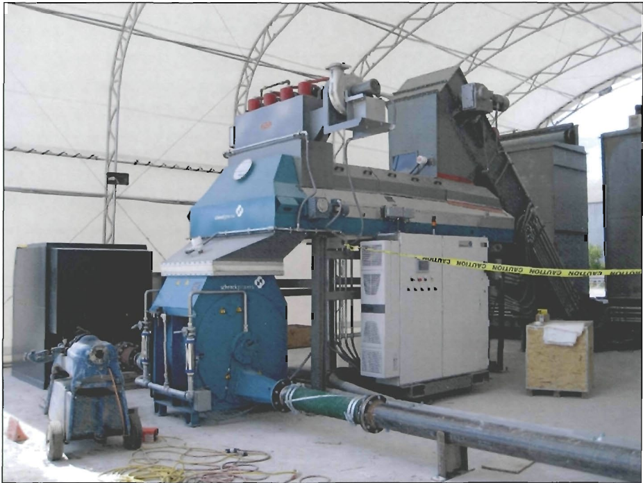
FIGURE 5. PNEUMATIC BLOWER FROM METERING SYSTEM TO INJECTION PORTHOLE.
