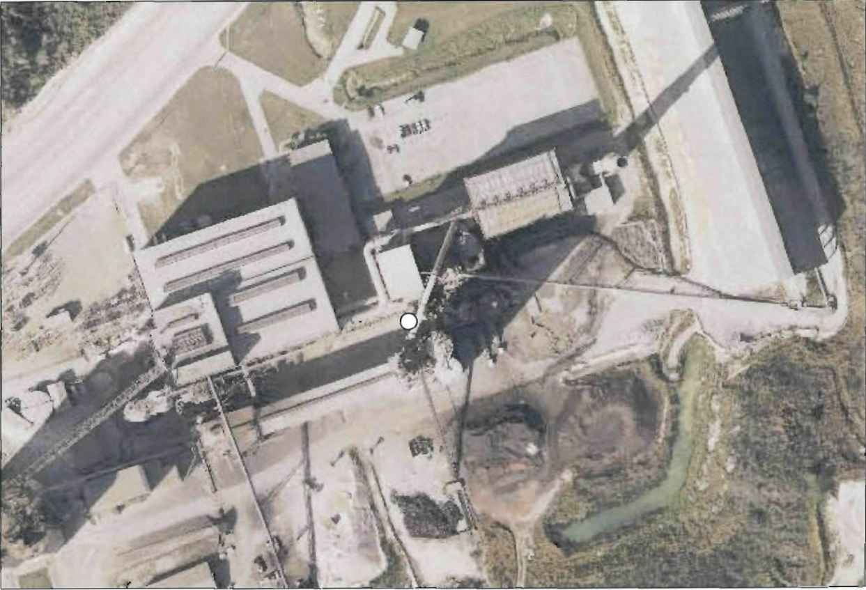
FIGURE 7. LOCATION OF THE PROCESSING AREA NEXT TO THE KILN 2 PRECALCINER.
