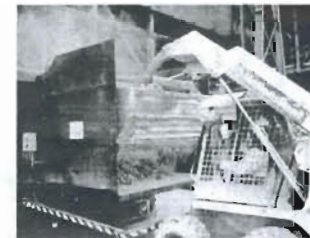
Feed: Dust is fed to conveying equipment using a bobcat.
