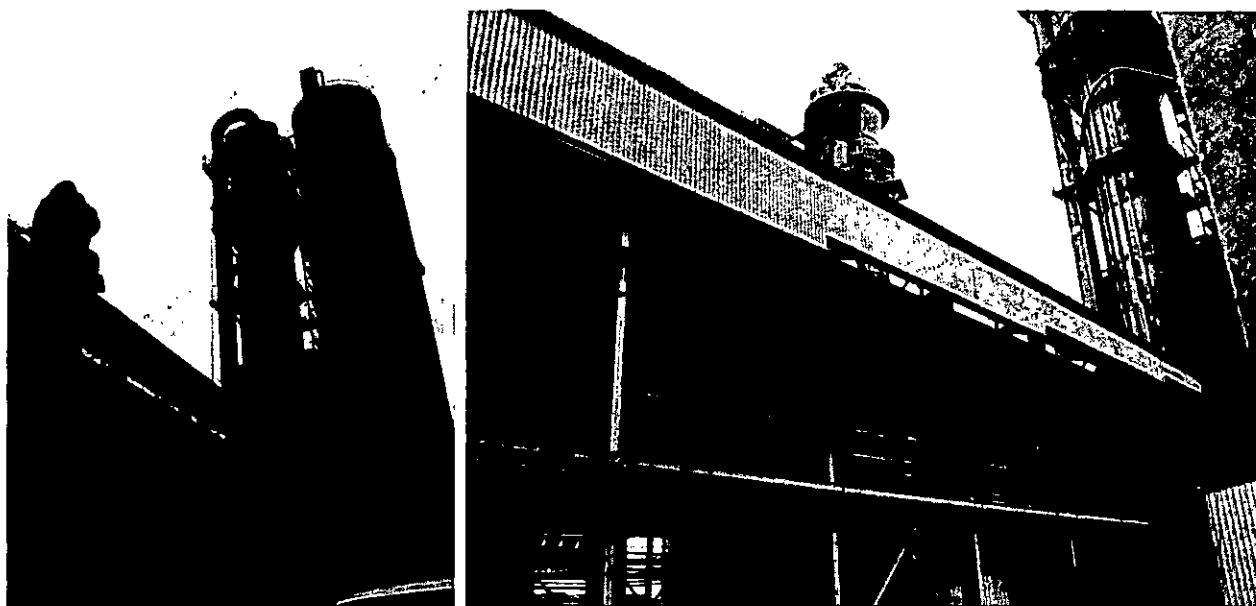
Figure 2. Polysius GEPOL Preheater Kiln at CEMEX North Brooksville Plant
