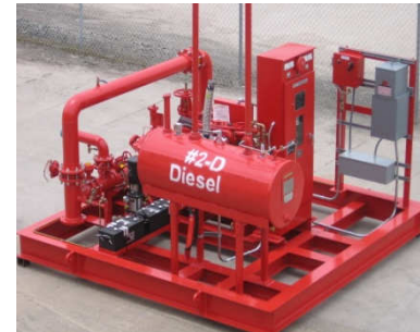
EMERGENCY FIRE WATER PUMP
