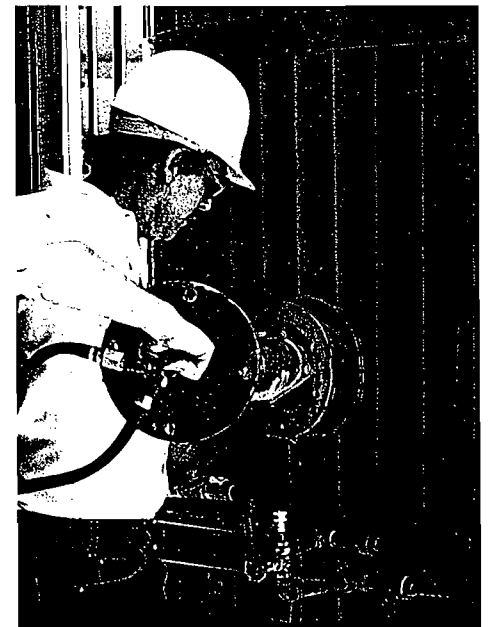
Easy removal and replacement of the lance assemblies facilitate maintenance.
