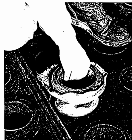
28. Compression band is attached at bottom of cage.
