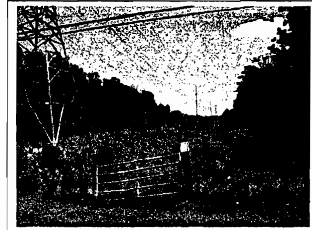
View of Existing JEA Transmission Line Located on Subject Site
