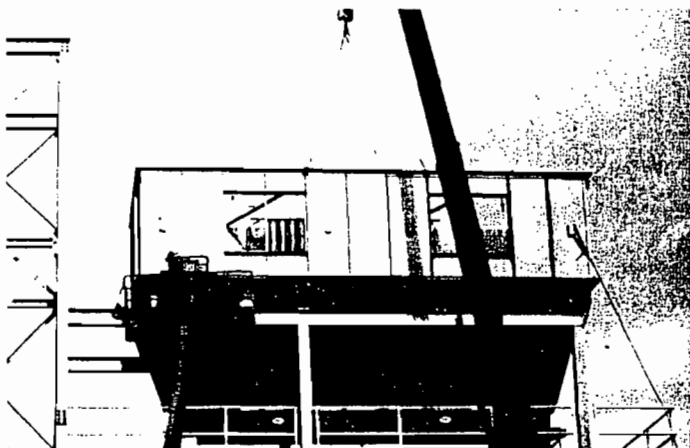
Housing is set in place on hopper.
