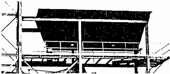
Hopper is placed on support steel.
