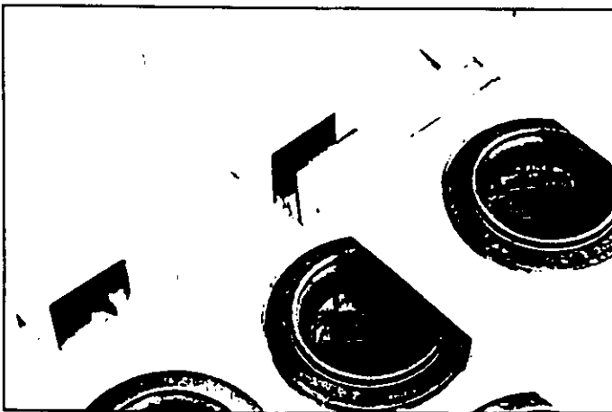
Step 5 The header pipes are easily installed by sliding the indexed bracket into the bracket.
