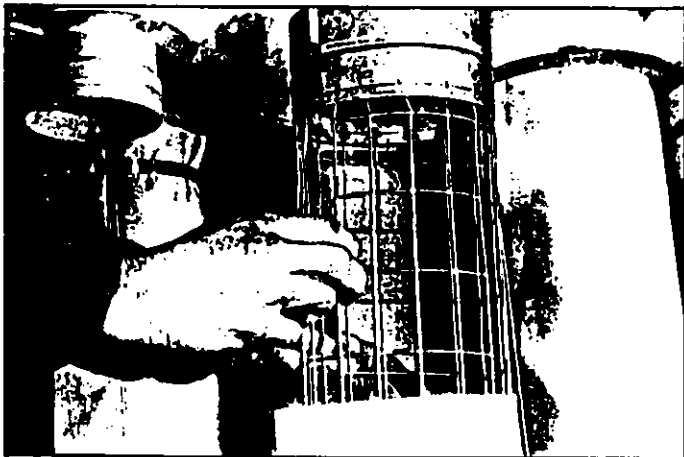
Step 1 The cage is inserted into the full length of the bag.
