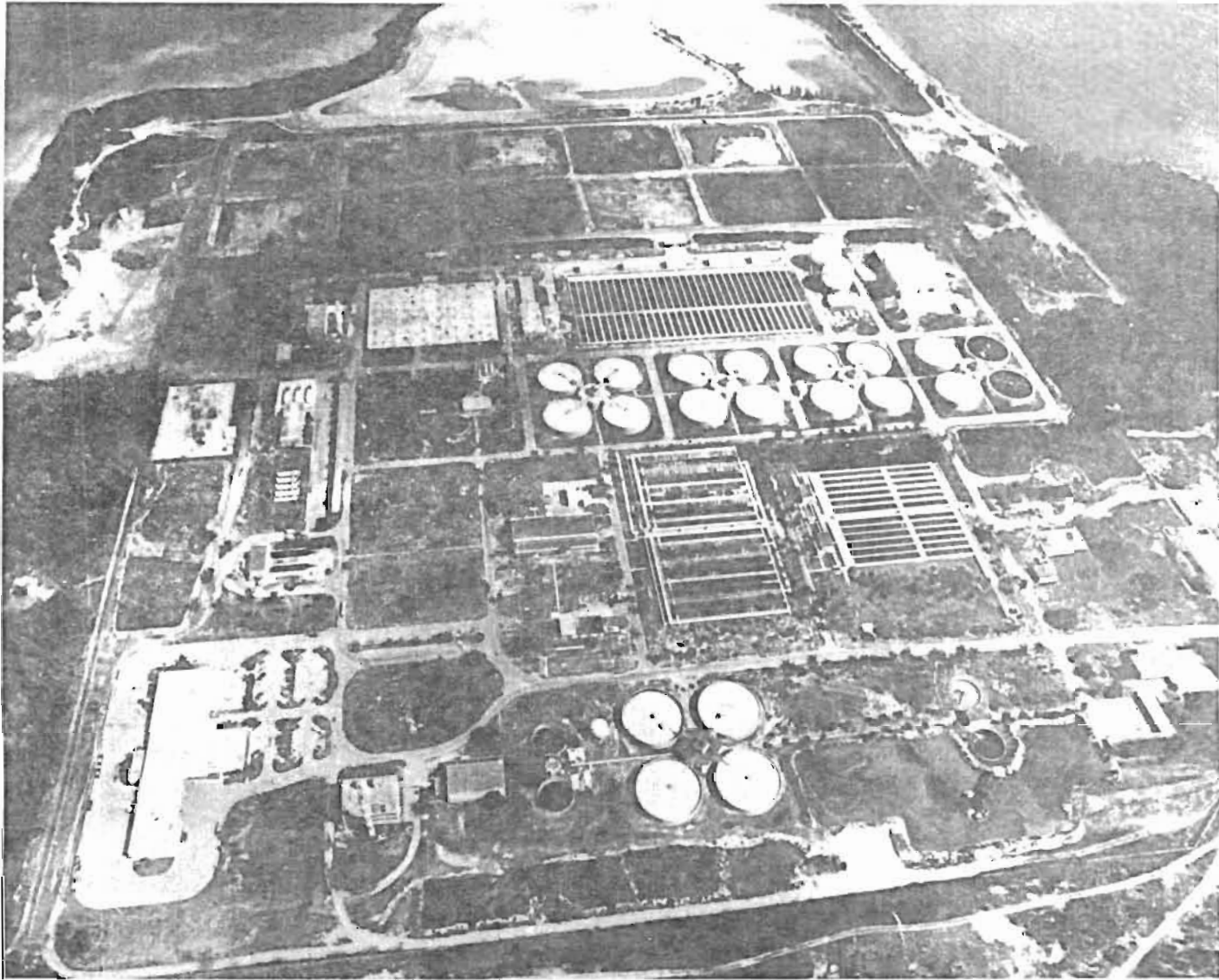
CENTRAL DISTRICT WASTEWATER TREATMENT PLANT - 1982
