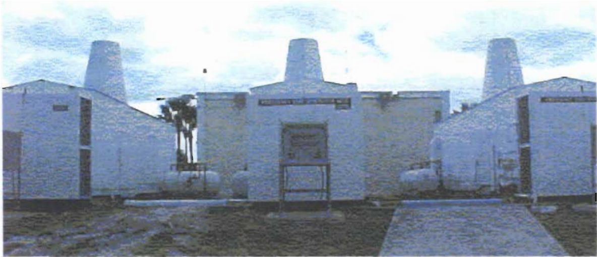
Figure 3-1 - Photograph of the Existing EMD Units at the Central District WWTP
