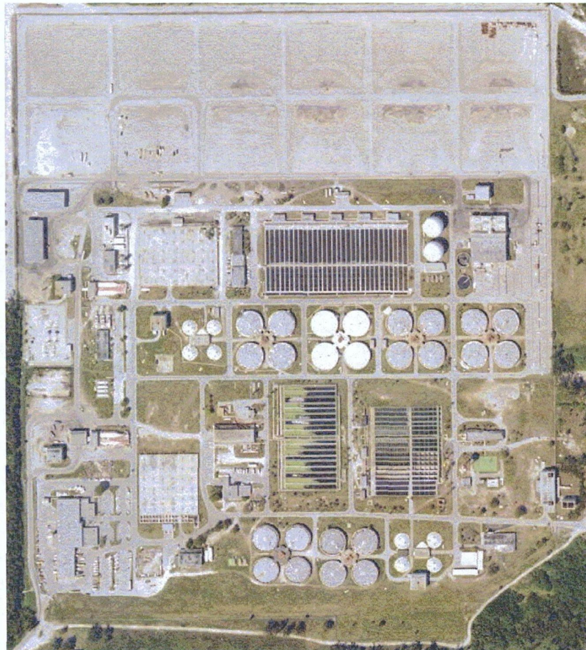
Figure 2-1 Aerial Photograph of the Central District Wastewater Treatment Plant
