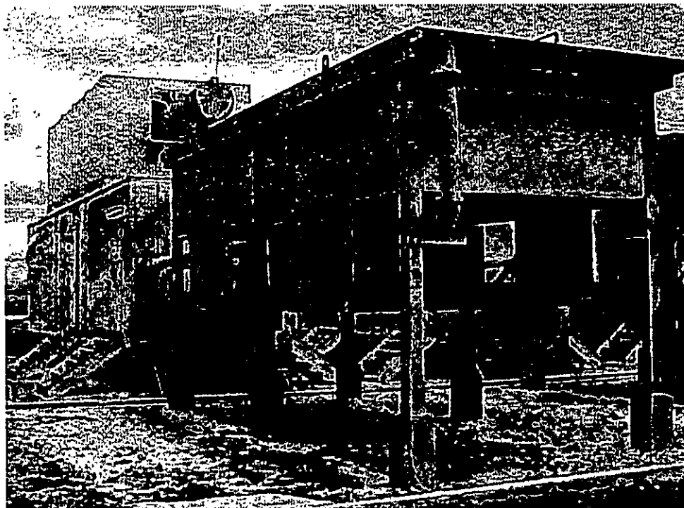
Figure 3-2 - EMD Model 20-645F4B Unit with External Radiator
