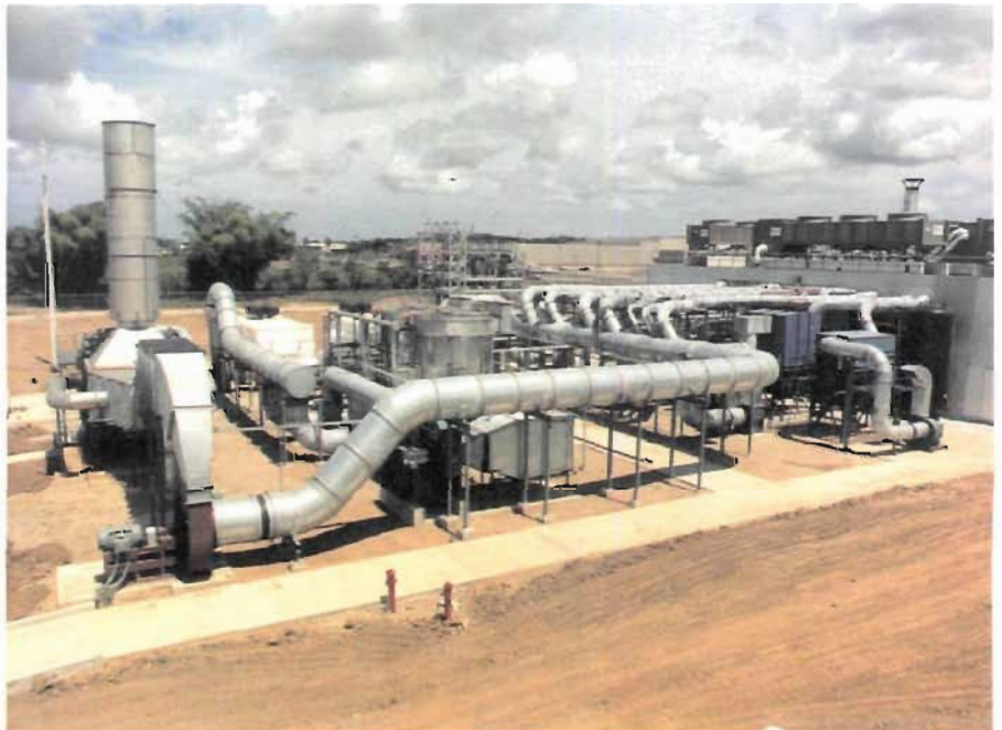
Key Pharmaceuticals needed to install a solvent recovery system and a catalytic incinerator to treat both chlorinated and non-chlorinated solvents
