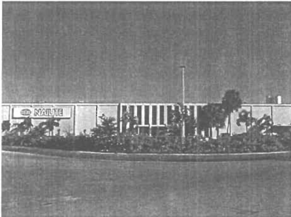
Nailite Vinyl Panel Manufacturing Facility
