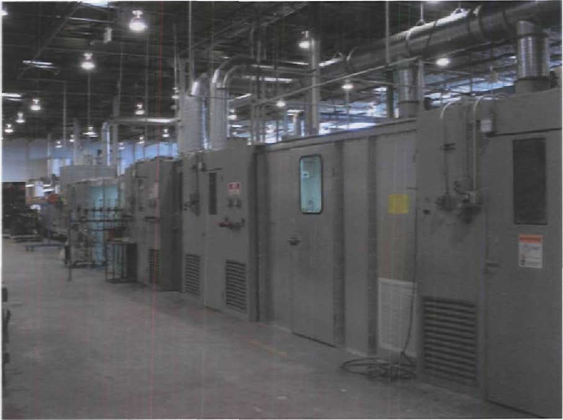
Paint line No. 1- loading end.
