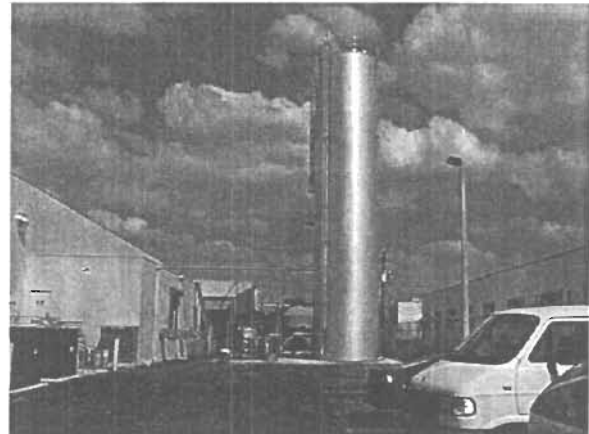
Raw Material (Polypropylene) Storage
