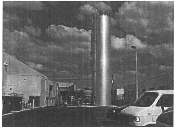
Raw Material (Polypropylene) Storage
