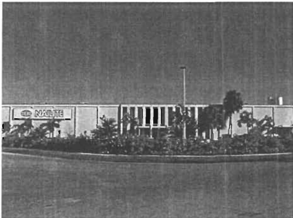
Nailite Vinyl Panel Manufacturing Facility
