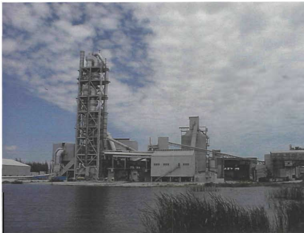
CSR Rinker Modernized Dry Process Cement Plant in Miami, Florida
