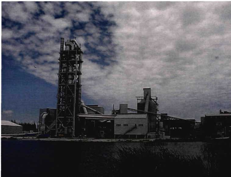
Rinker Modernized Dry Process Cement Plant in Miami, Florida
