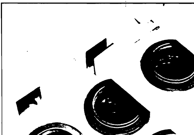
Step 5 The header pipes are easily installed by sliding the indexed end into the bracket.
