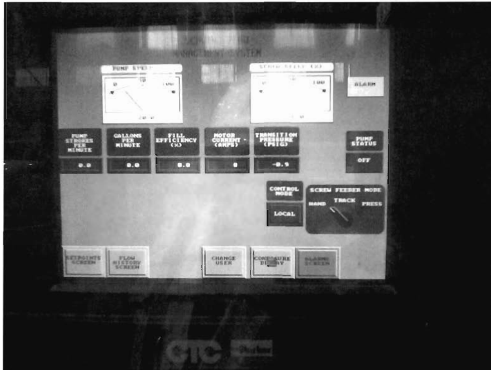
Figure 9 – Screw/Pump Control Screen
