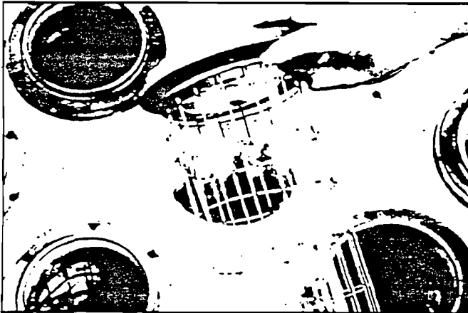
Step 3 Snap band with high profile lip seals secure the bag to the tube sheet.
